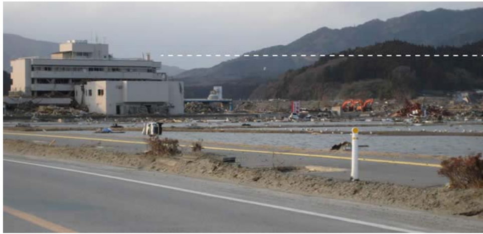
Figure 1. Takata Hospital, Rikuzentakata City, 2 April 2011. The tsunami reached to the level of the broken line.
